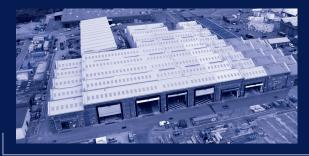
The site includes 27 support bays, giving some 51,416m2 of manufacturing space with crane capacity up to 35 tonnes.
